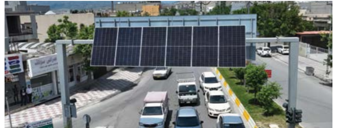
Traffic lights at an intersection in Erbil that are powered by solar energy
